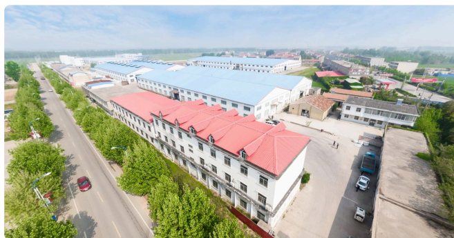
Hechuang manufacturing facility, Donghai County
